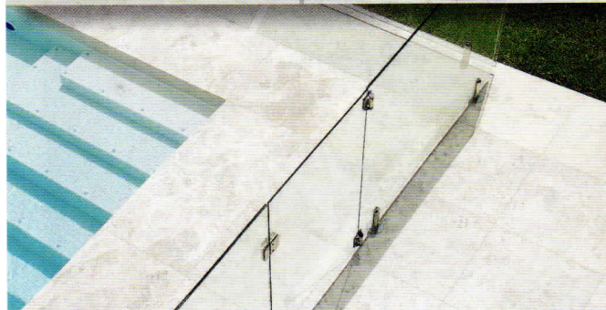
This pool is fully tiled in GCR 305 White Crystal Pearl Blend 20mm glass mosaics. Silver Marble 610 x 610 x 30mm Square Edge Coping has been used on the edge of the pool to match the 610 x 610mm tiles used for the surround paving.
