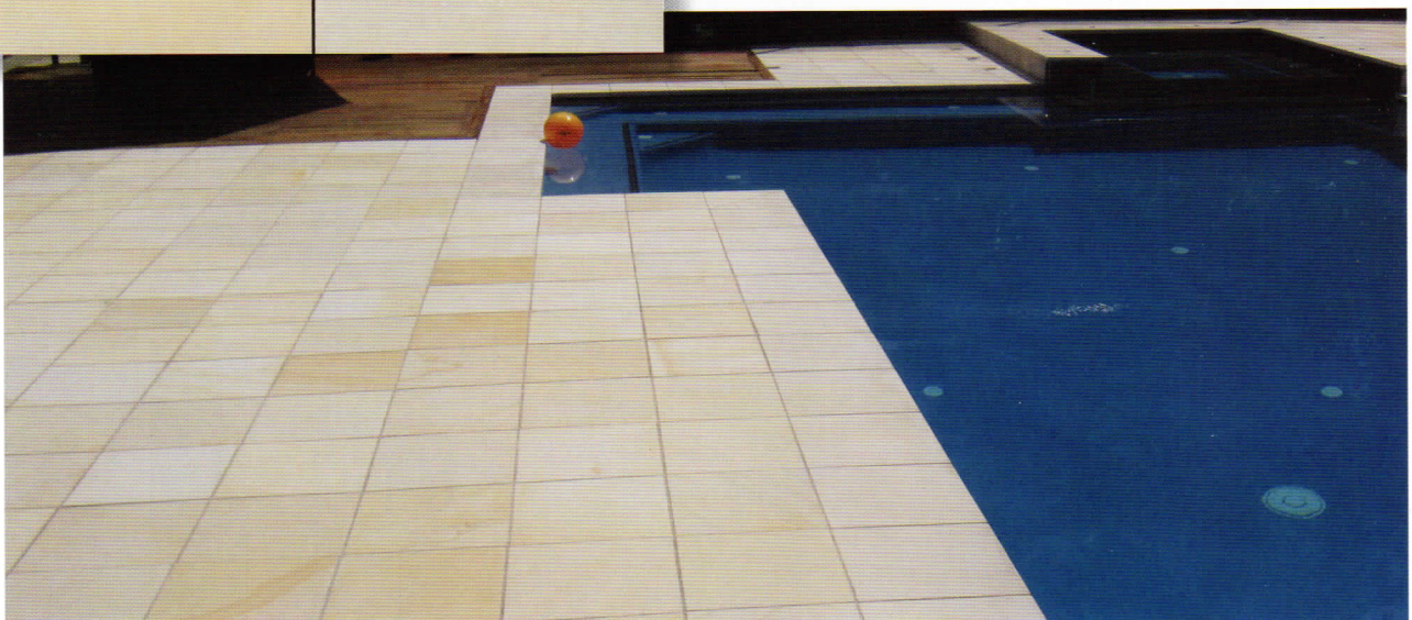
Rebated Square Edge 400 x 400 x 40/20mm has been used on the coping of this pool. The matching 400 x 400 x 15mm tiles have been used for the surround paving.
